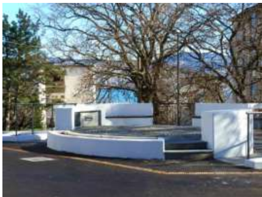
Figure 11: Completed, new square in Borgo Zindis
